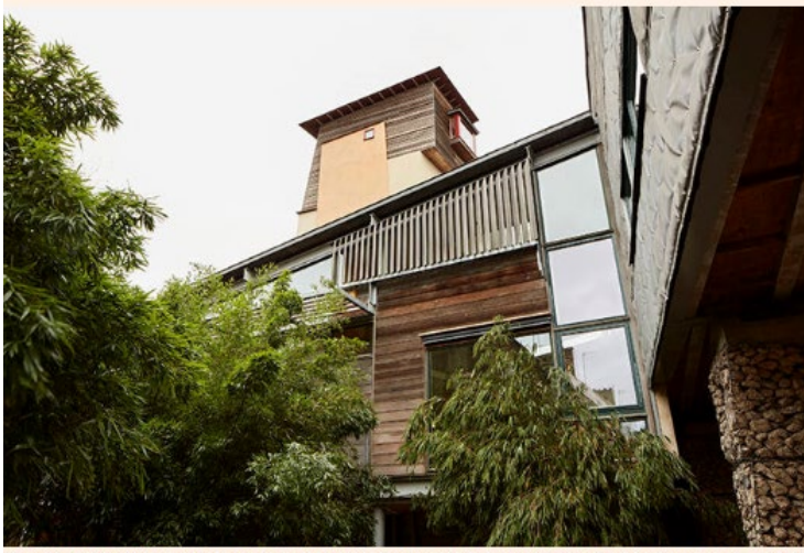
The exterior of Sarah Wigglesworth's house: by 2030, one in five people in the UK will be aged 65 or over; those over 85 — 1.6m as of 2016 — are expected to double by 2041 and treble by 2066 © Thom Atkinson for the FT
