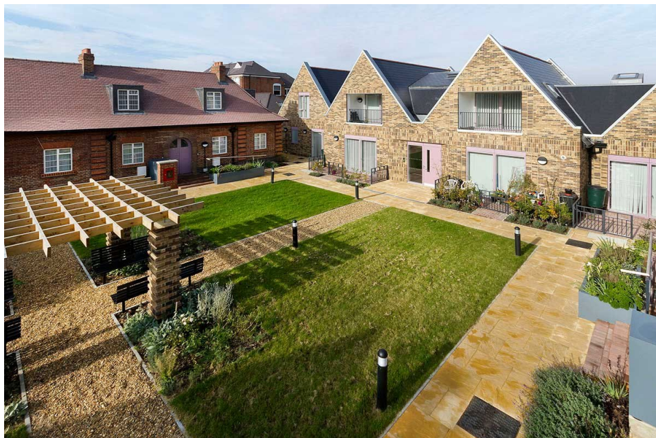
Thrale Almshouses in Streatham. The scheme consists of 17 affordable homes (picture: Robert Greshoff/BPTW)
