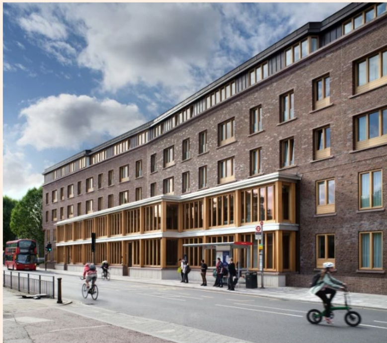
The contemporary exterior of Appleby Blue, which has 51 one-bedroom apartments and six two-bedroom flats © Philip Vile/Witherford Watson Mann Architects
