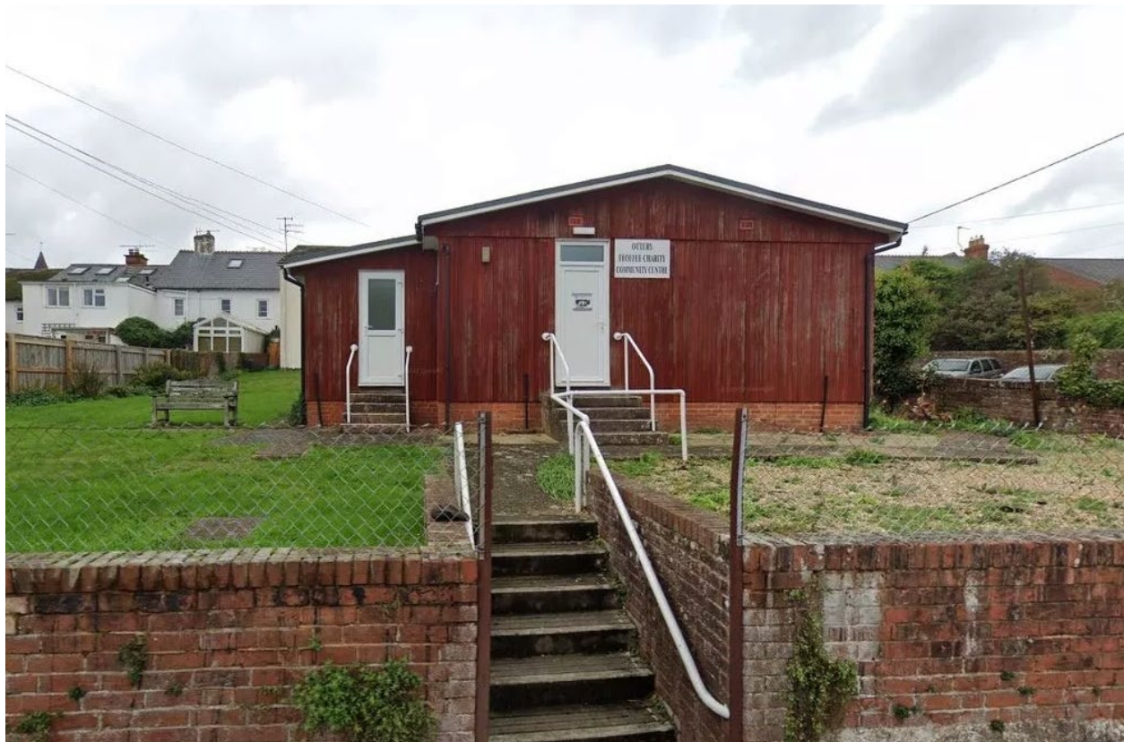
The old day centre before demolition.
