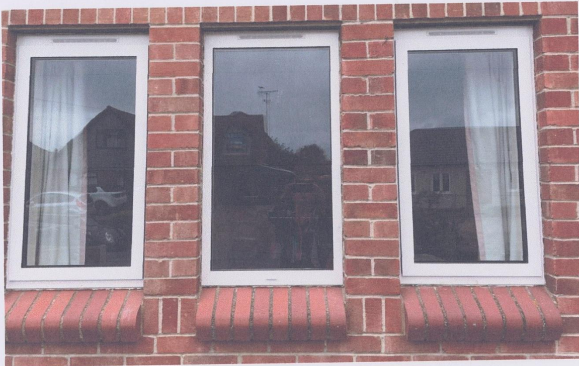
New Bedroom Windows (External)
